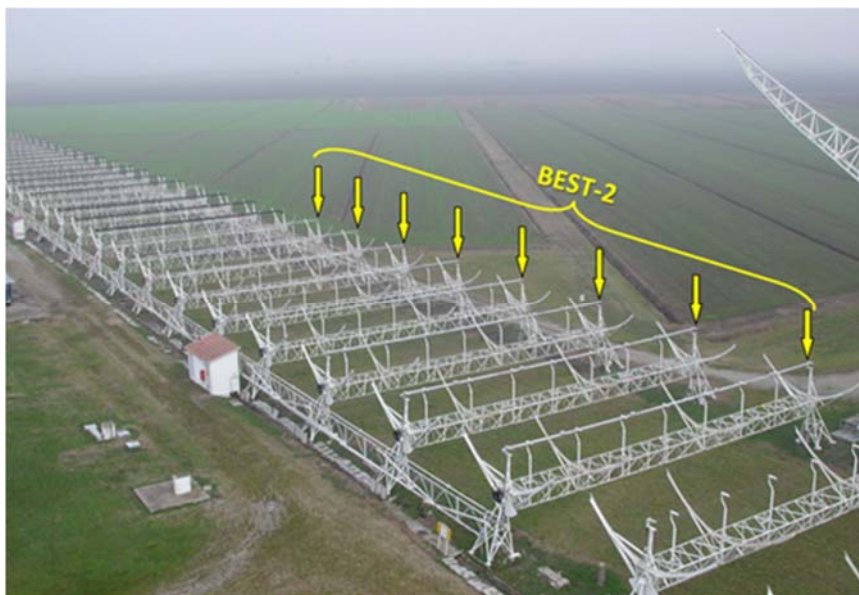
Figure 4.1. BEST-2 elements inside the N-S arm of the Northern Cross.
